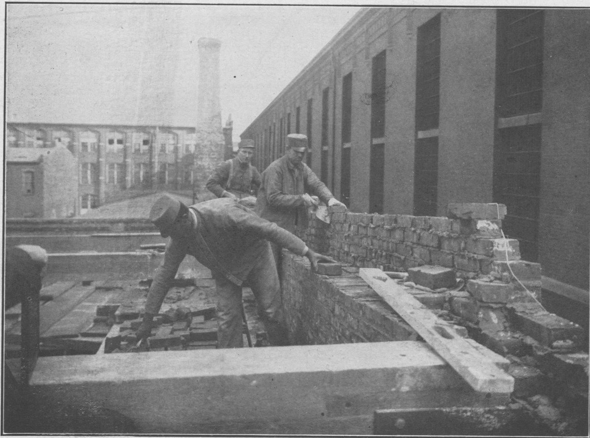
MASONS AT WORK
