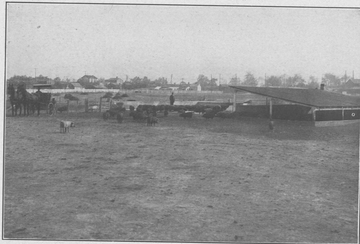
HOG YARD AND SANITARY SHED
