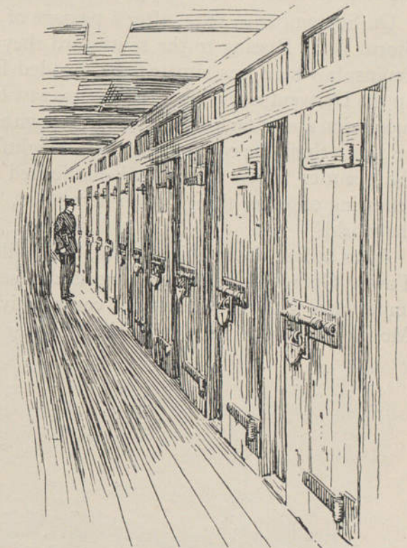
CELLS BETWEEN DECKS
