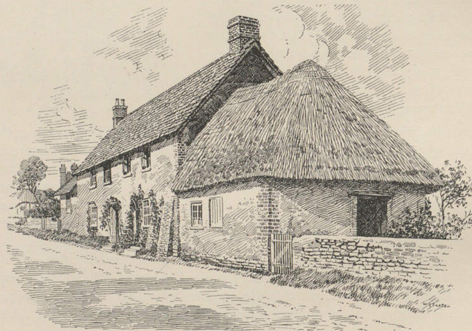
STANDFIELD'S COTTAGE AT TOLPUDDLE
