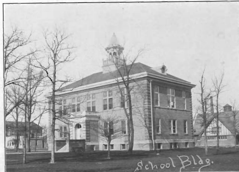
SCHOOL BUILDING WITH CHAPEL AT THE RIGHT ILLINOIS TRAINING SCHOOL FOR GIRLS, GENEVA
