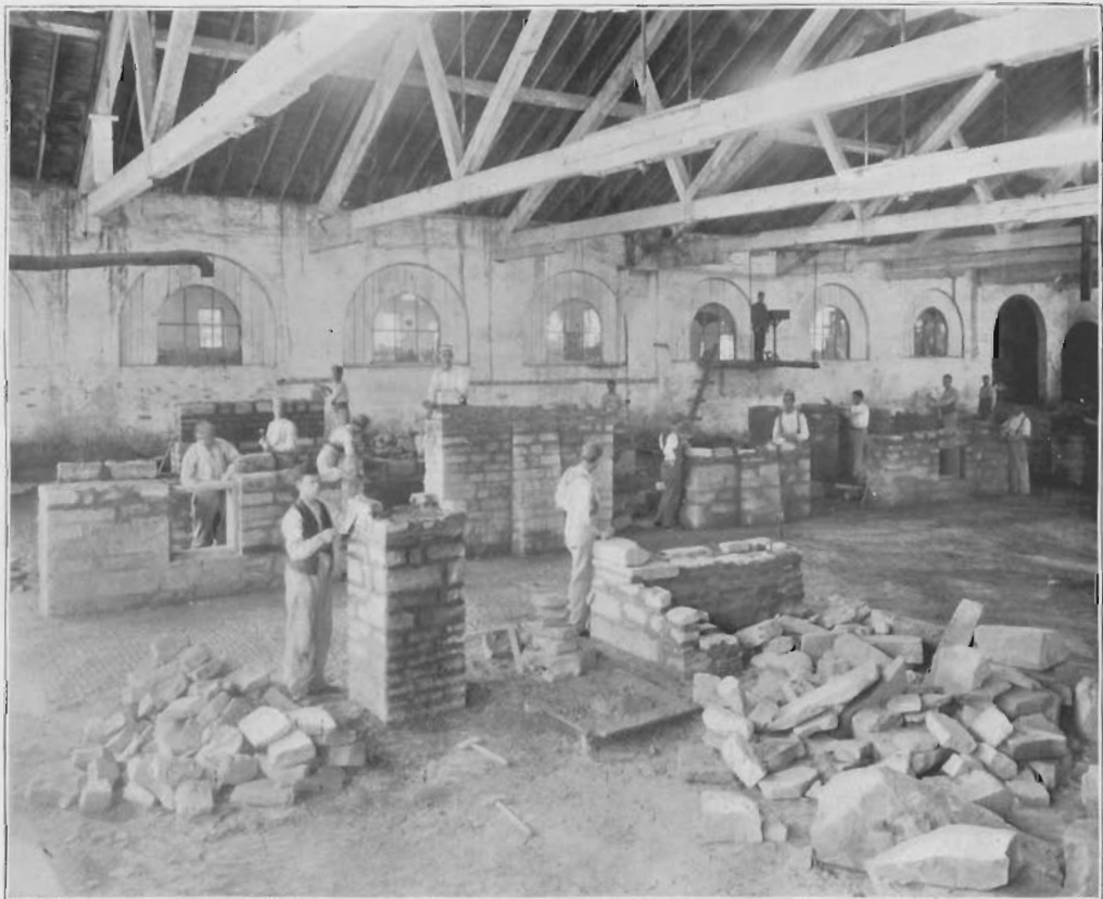
ELMIRA REFORMATORY. BRICKLAYING AND MASONRY.
